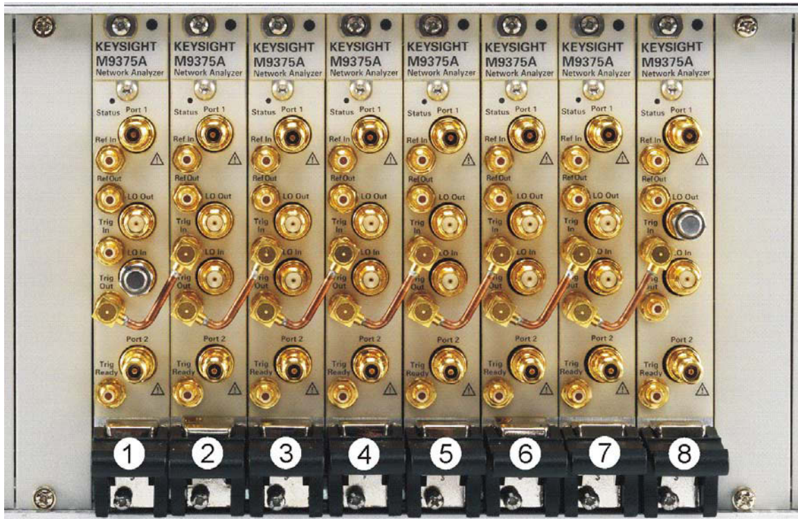
Figure 1-7 Installing Semi-Rigid Cable M9370-20018
